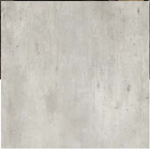
2204F00-WF CRACKED CEMENT
